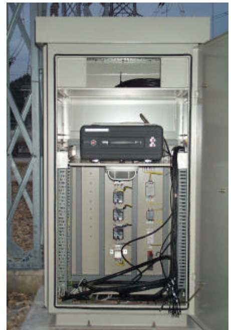
On-Site installed PD Monitoring System LDWD-6
