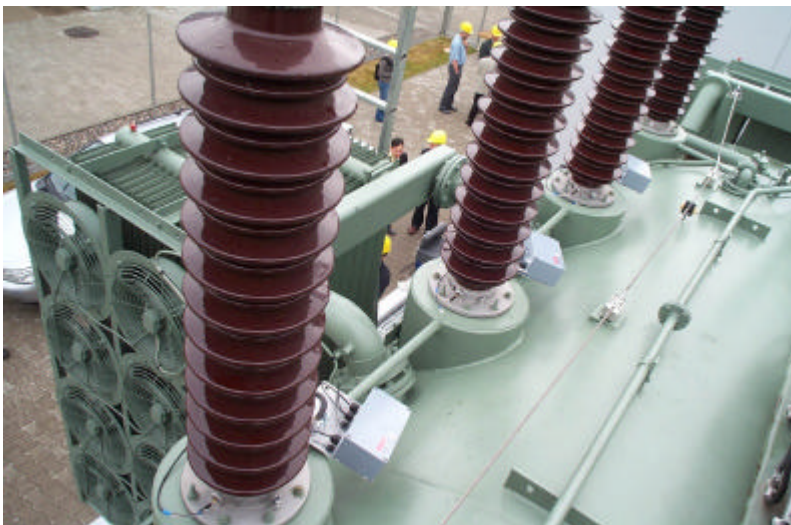
PD coupling units installed on a power transformer
