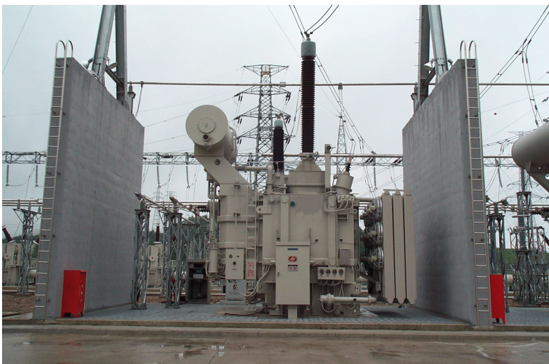
Monitored 345 kV power transformer
